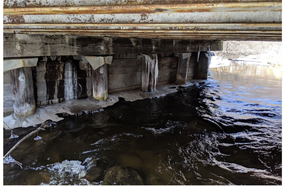
Under 20' Structure, Barron County
