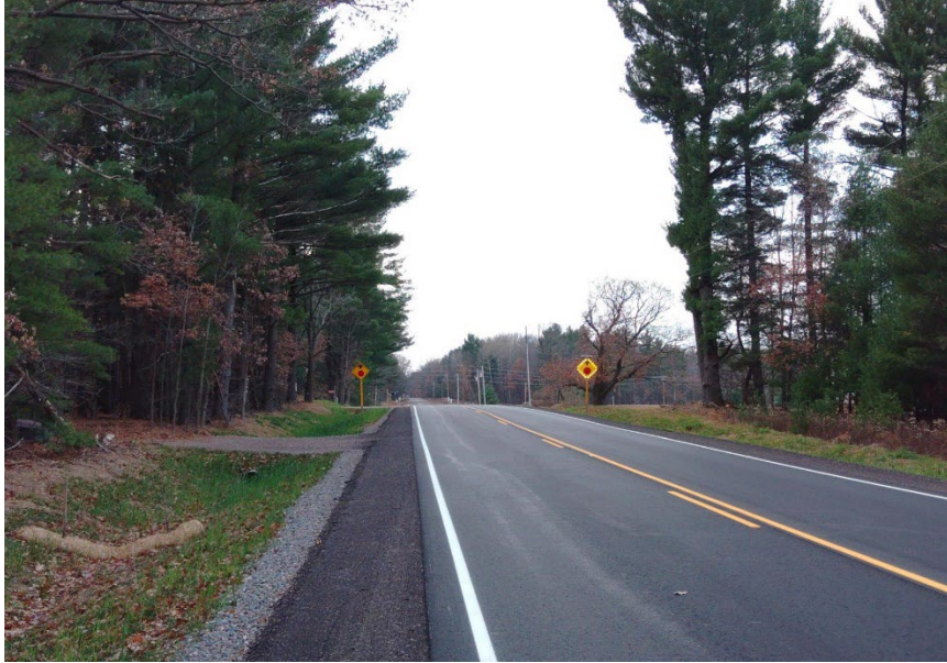
Wood Co. Highway Redone with LRIP-S
